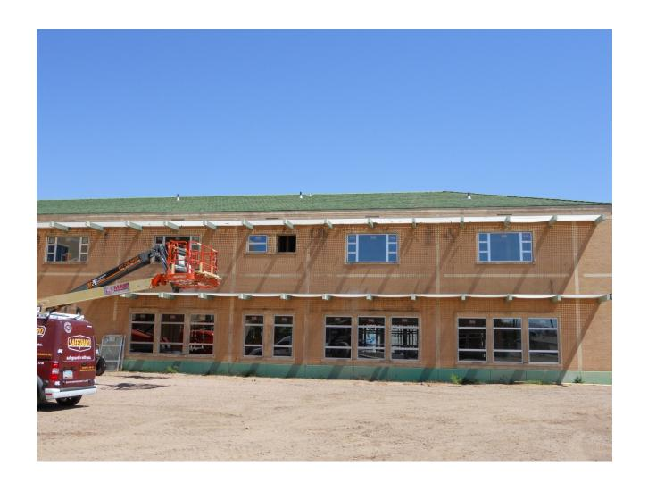
Original clay tile replaced and new windows (approved by both SHPO and NPS) being installed.
