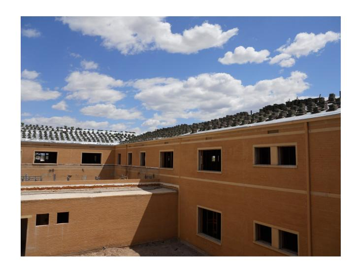
Every single original clay tile was removed and radiant barrier added to meet ADOH Sustainable Development standards for energy efficiency.
